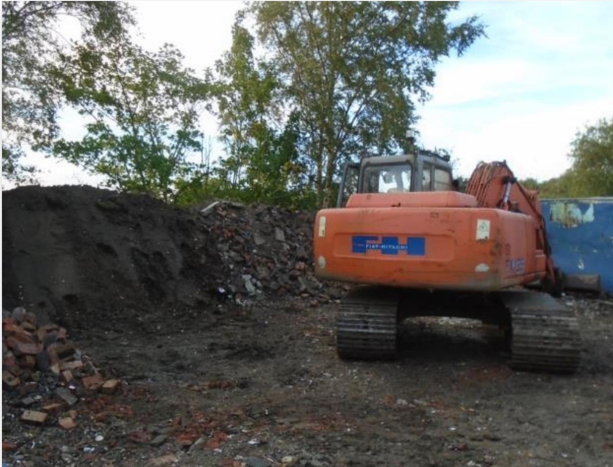
Aggregate/soil storage area
