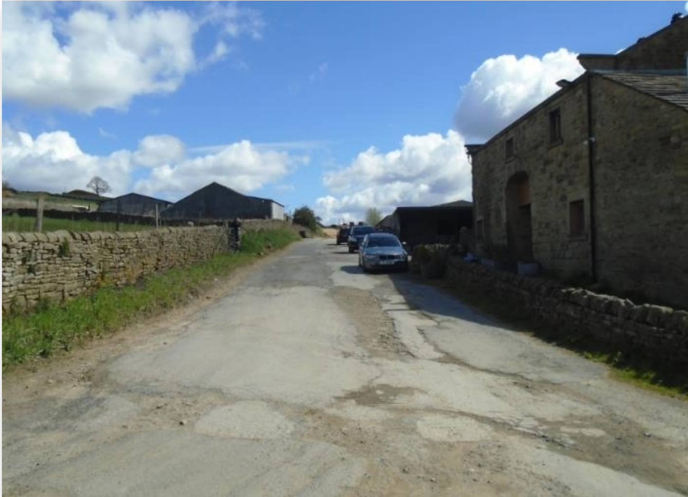
Crawshaw Lane at the junction with Southfield Lane
